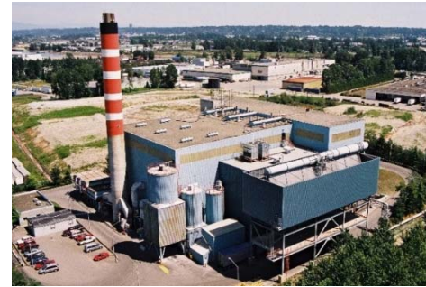
Photo 4: Burnaby WTE Facility.
