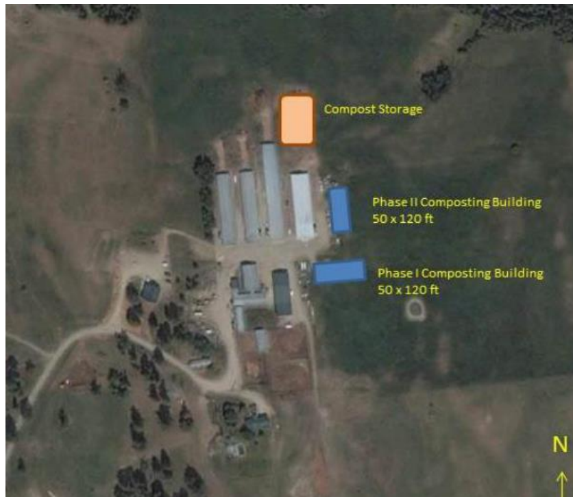
Figure 4-2: Phase 1 and 2 Compost Building and Storage Area at Spa Hill Farm
