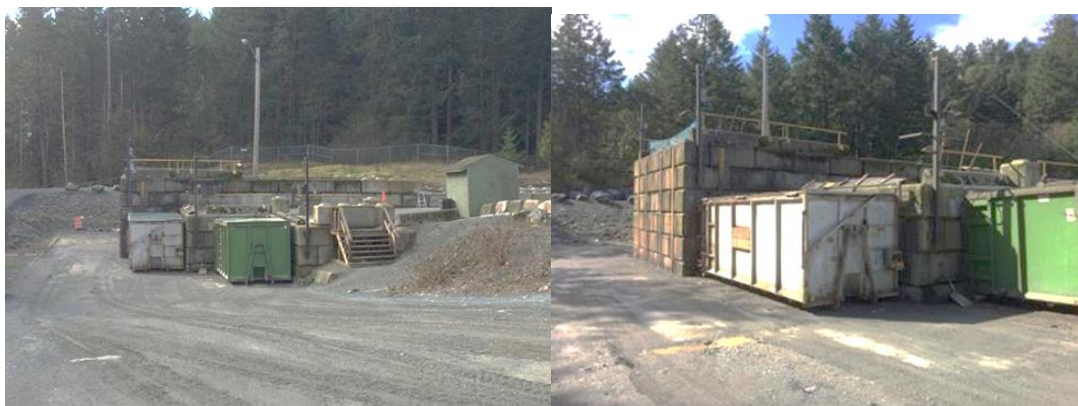
Figure 4-3: Hartland Landfill Food Waste Transfer Site
